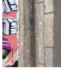
Heritage stone gutters
